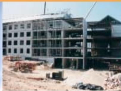
Hilltop Residence Hall Storrs, CT
